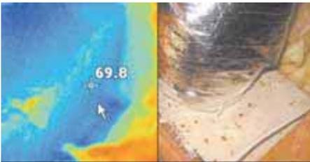
Figure 2: Thermal image (left) and visible light image of duct boot under insulation. Note surface temperature reading on thermal image.
