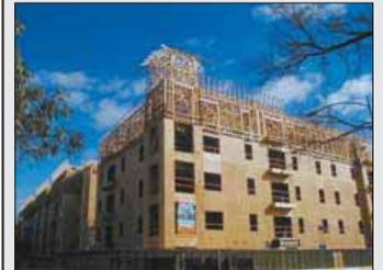
Stick frame multi-story construction in Austin, TX. Note plywood (engineered wood) sheathing.
