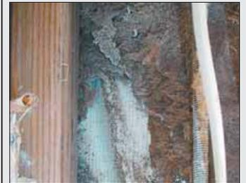
Visible building wrap and back of stucco after OSB disintegrated. Cause: low volume window leak. IET photo.
